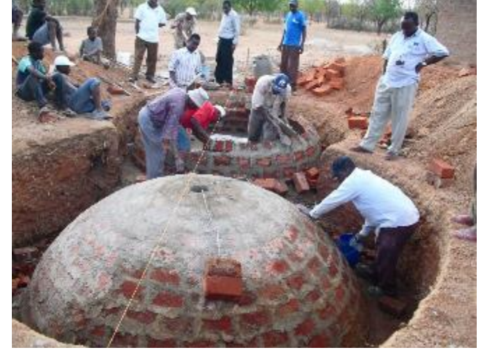
Fixed dome biogas digester
